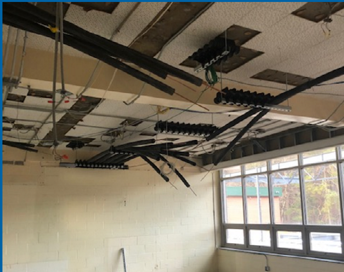
NE Wing Mechanical VRF Rough-In
