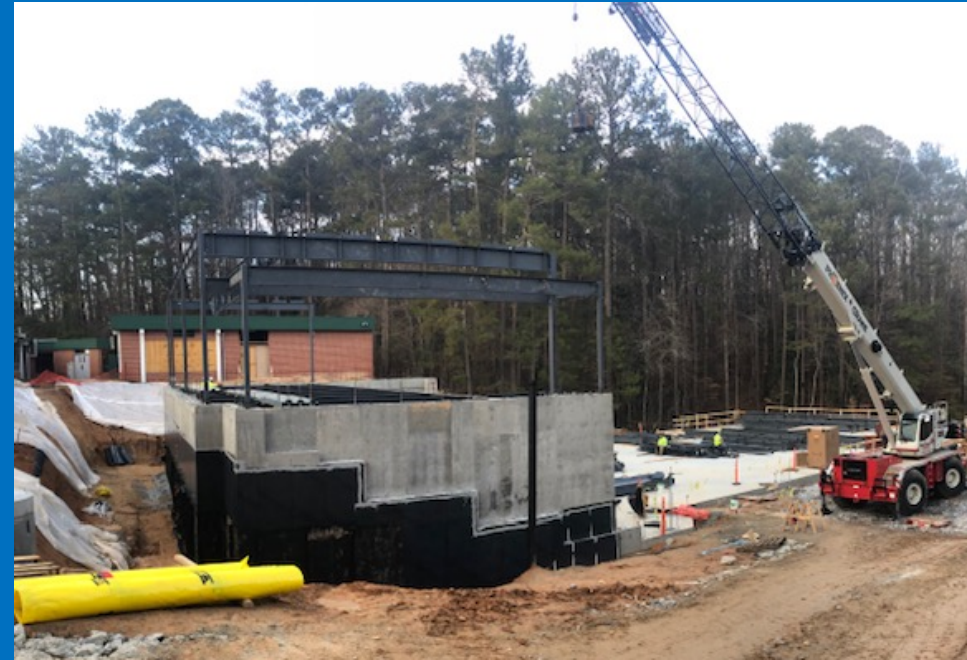
Start of Gymnasium Steel Erection
