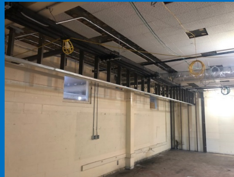
Interior Metal Framing at Renovation
